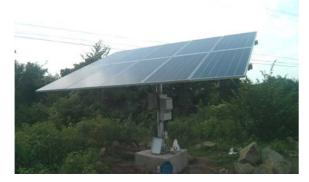
Smart Tracker for PV panels for improved efficiency.
